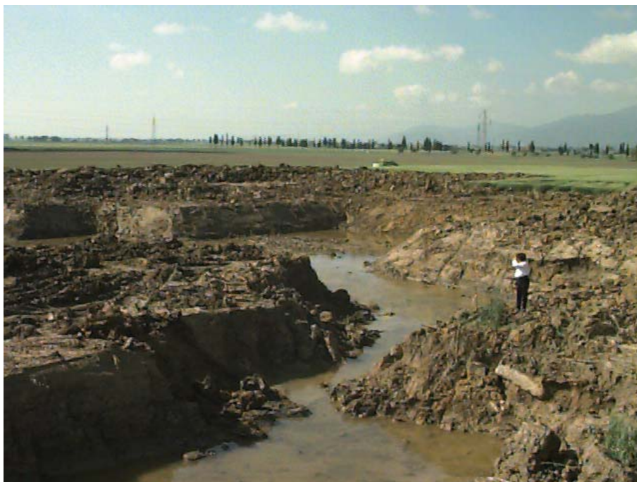
The site of the central building shortly after start of the construction works
