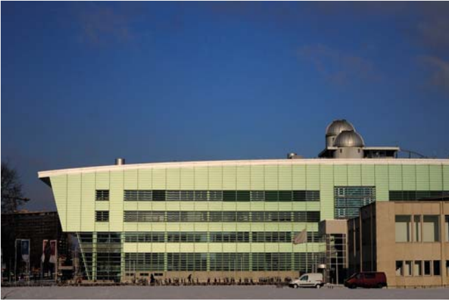
Fig. 1: The building hosting the Department of Astrophysics at Radboud University
